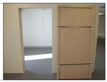
**VERY IMPORTANT** (Floor Preparation): Ensure that the floor under the door slab is flat and level. You may install a flat, level, and smooth threshold. If the existing floor is not flat, level, and smooth-the bottom door seal will not perform properly. DO NOT raise the hinge side of the jamb off of the floor. The factory undercut of the door is set to the proper height.
