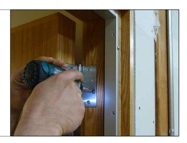
INSTALL TIP, IF SEAL REMOVAL IS NEEDED TO MAKE CONTACT INTO SOLID WOOD FRAMING: To remove the door seal, remove the screws going through the seal into the wood doorstops. Install long screws through the wood doorstops. Be sure to countersink the long screws so that the door seals rest flat on the wood doorstops. Reinstall the door seal with the screws previously removed from the seal.
